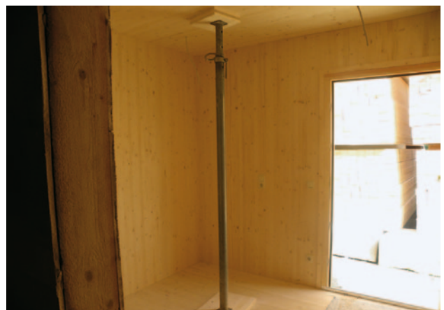
Fig. 2 - Etai support plancher
